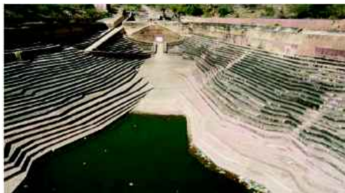
Fig. 16.6 : A Traditional Method of Rainwater Harvesting
